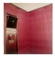
Follow the arrows as below for each panel (wall) with a cutout. Be sure to measure the cut-outs for each panel (wall) as they may differ in size.
